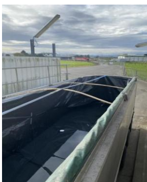
Figure 3: Bulk lines truck unit showing mechanical seals
